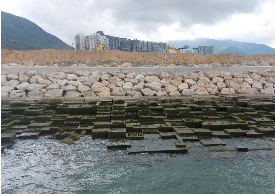
Photo 4 – Natural Rock Material/Planting for Artificial Seawall
