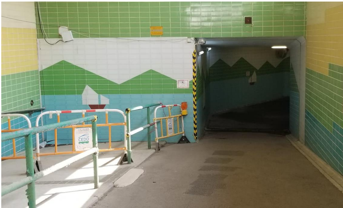
Photo 3 - Erection of site hoardings in unobtrusive colours
